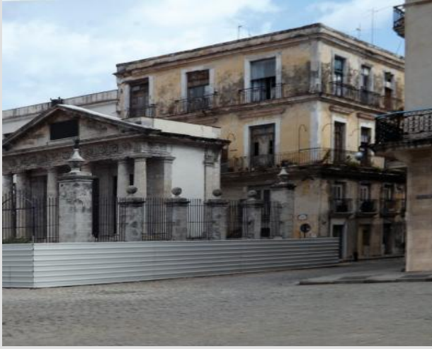
Many buildings in Havana appear in disrepair. Photo courtesy of K. K. Rhodes
